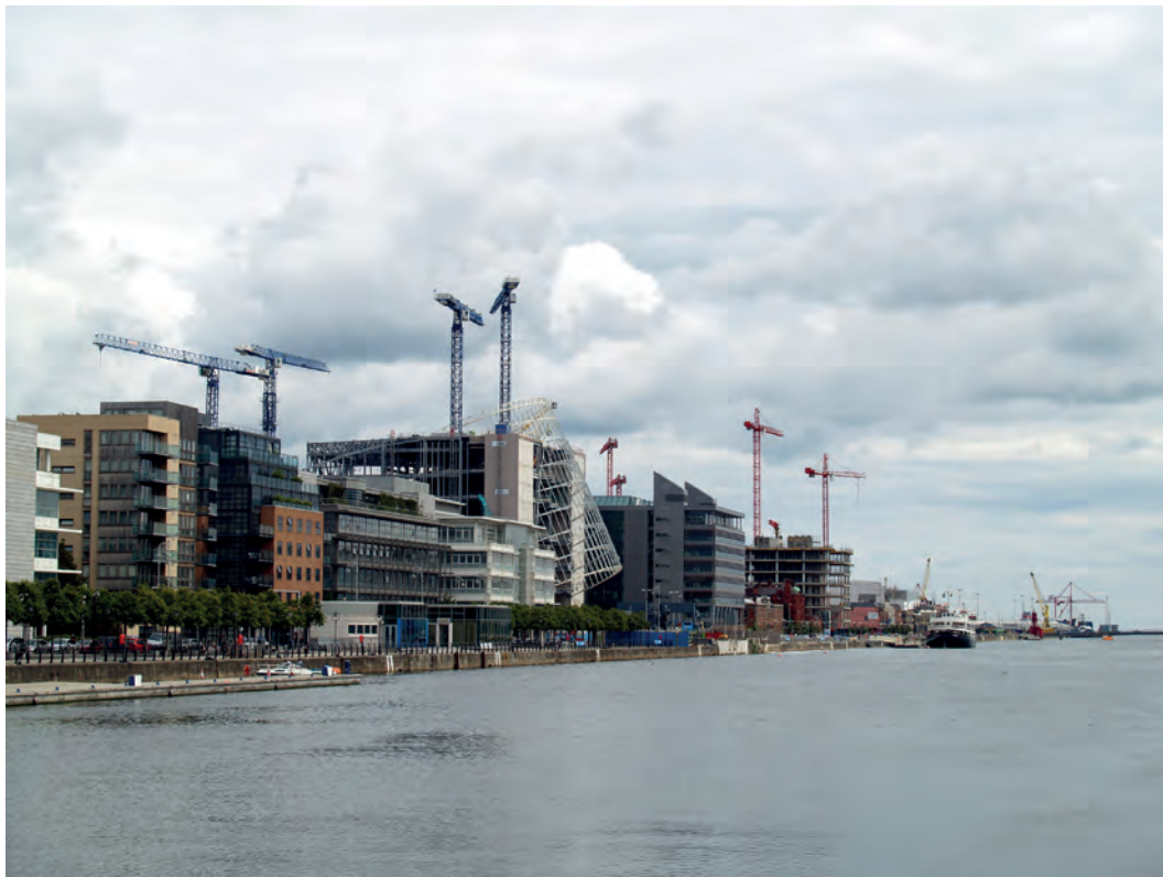
Figure 2 Urban regeneration scheme, Dublin, Ireland
